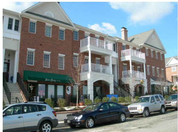
Eagleview TND: 3-story Live-Work Buildings enable vertical mixed use
