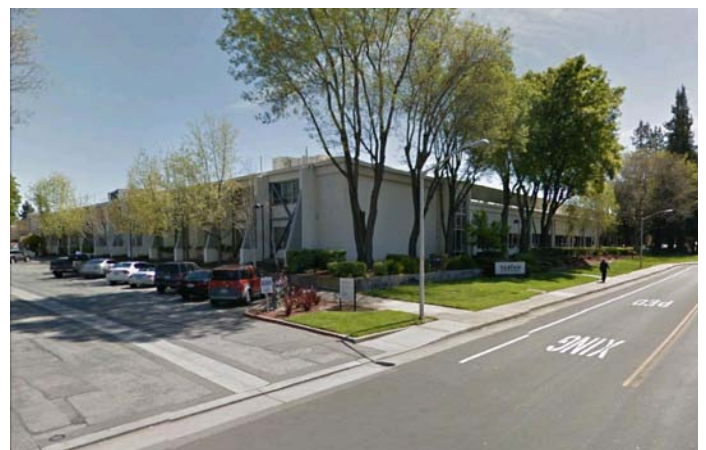
Stanford Research Park, Palo Alto, CA: Industrial building with parking to side.
