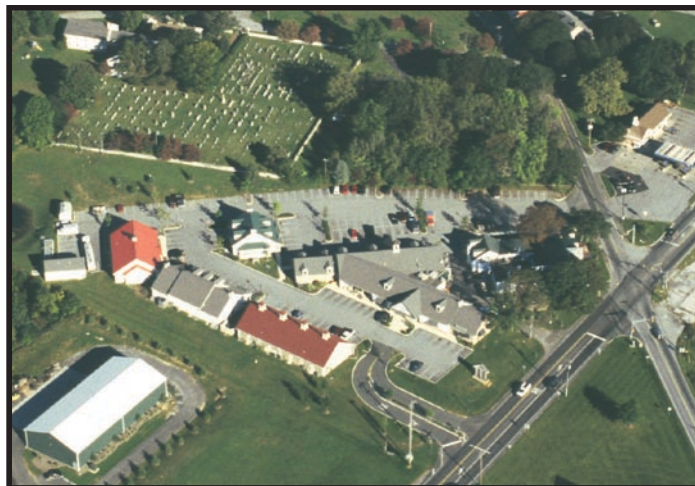
Angled Alignment of Buildings at Ludwig's Market
