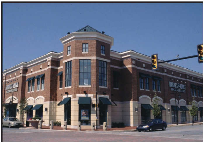
Two story building anchors corner
