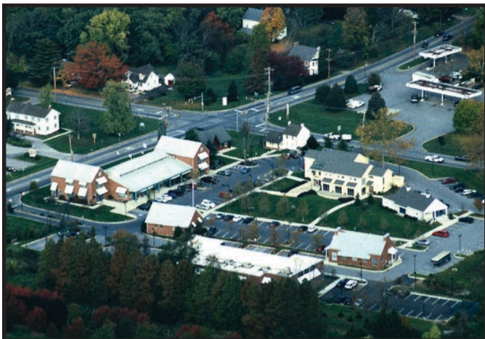
Aerial View of Site at Routes 82 & 926 in Chester County, PA
