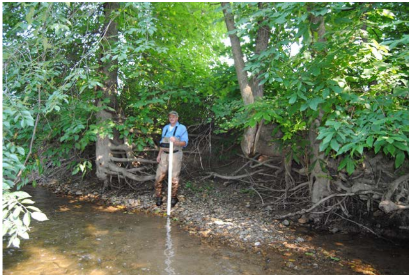
Photo 6 - Bank erosion and undermining of trees within Covered Bridge Park.
