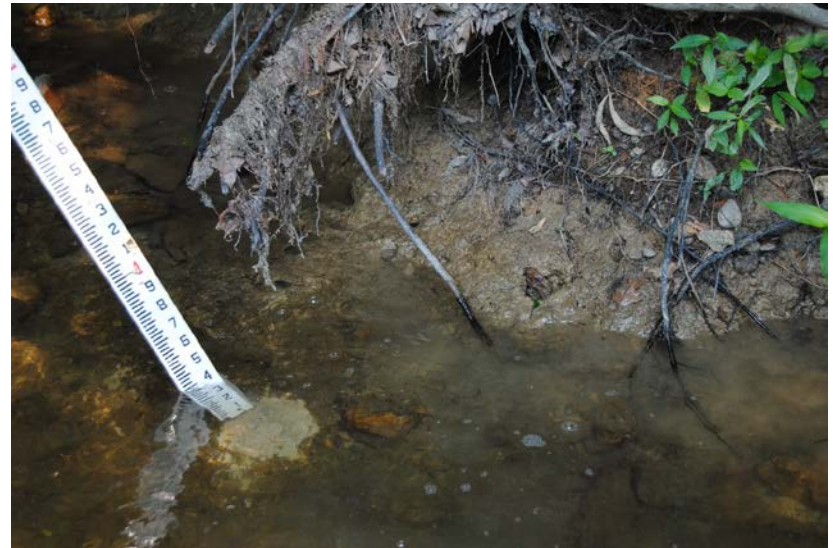
Photo 4 - Clay along the bank indicates that the stream is “perched” or raised from its historic elevation.
